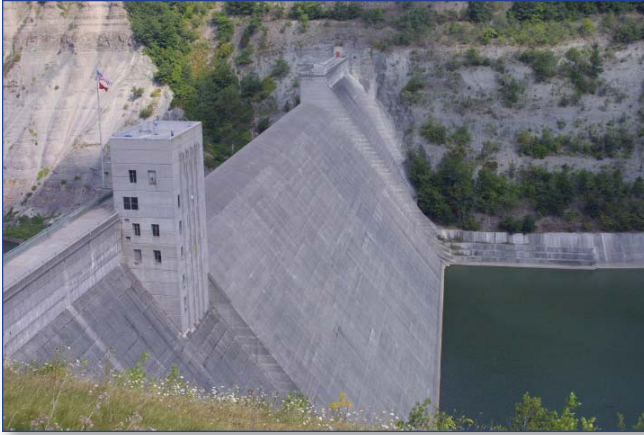
A hydroelectric facility located on the Genesee River in New York.
