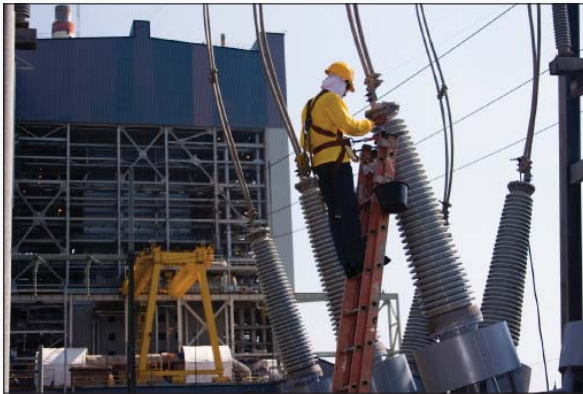
Worker at power station switchyard.
